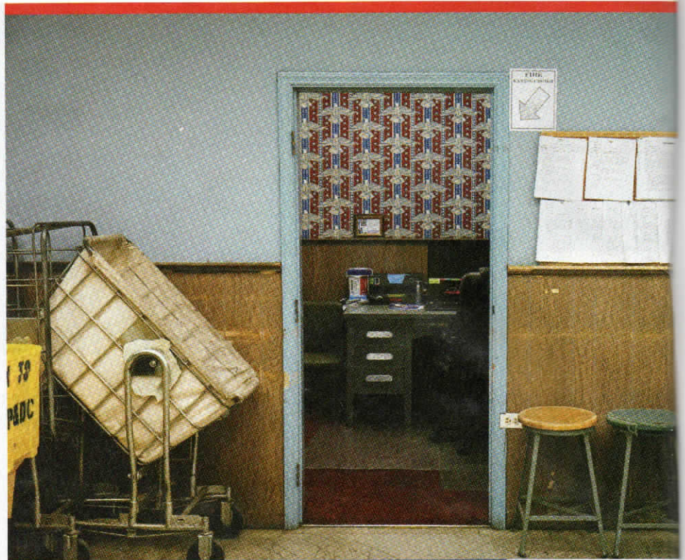
A post office in Comer, Ga., that DeJoy intends to upgrade
