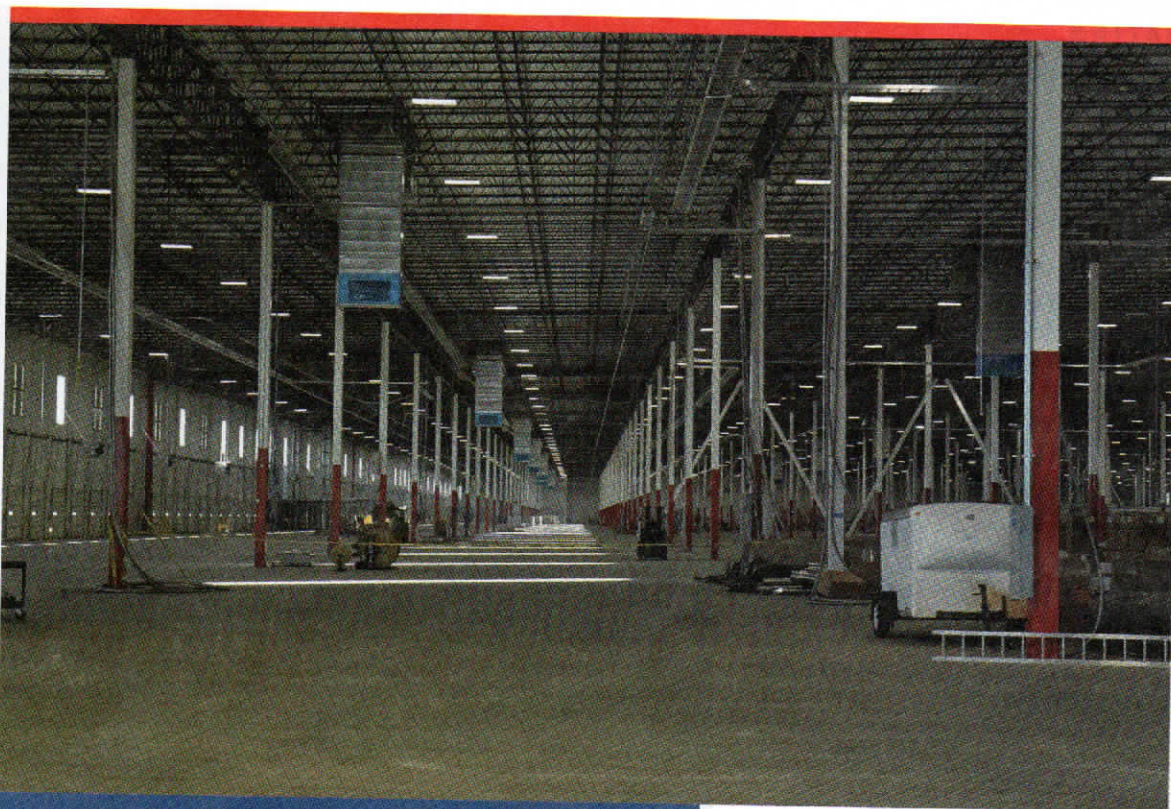
A new Postal Service processing facility in Palmetto, Ga.
